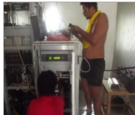
Repairing damaged telecommunication equipment in Nui
