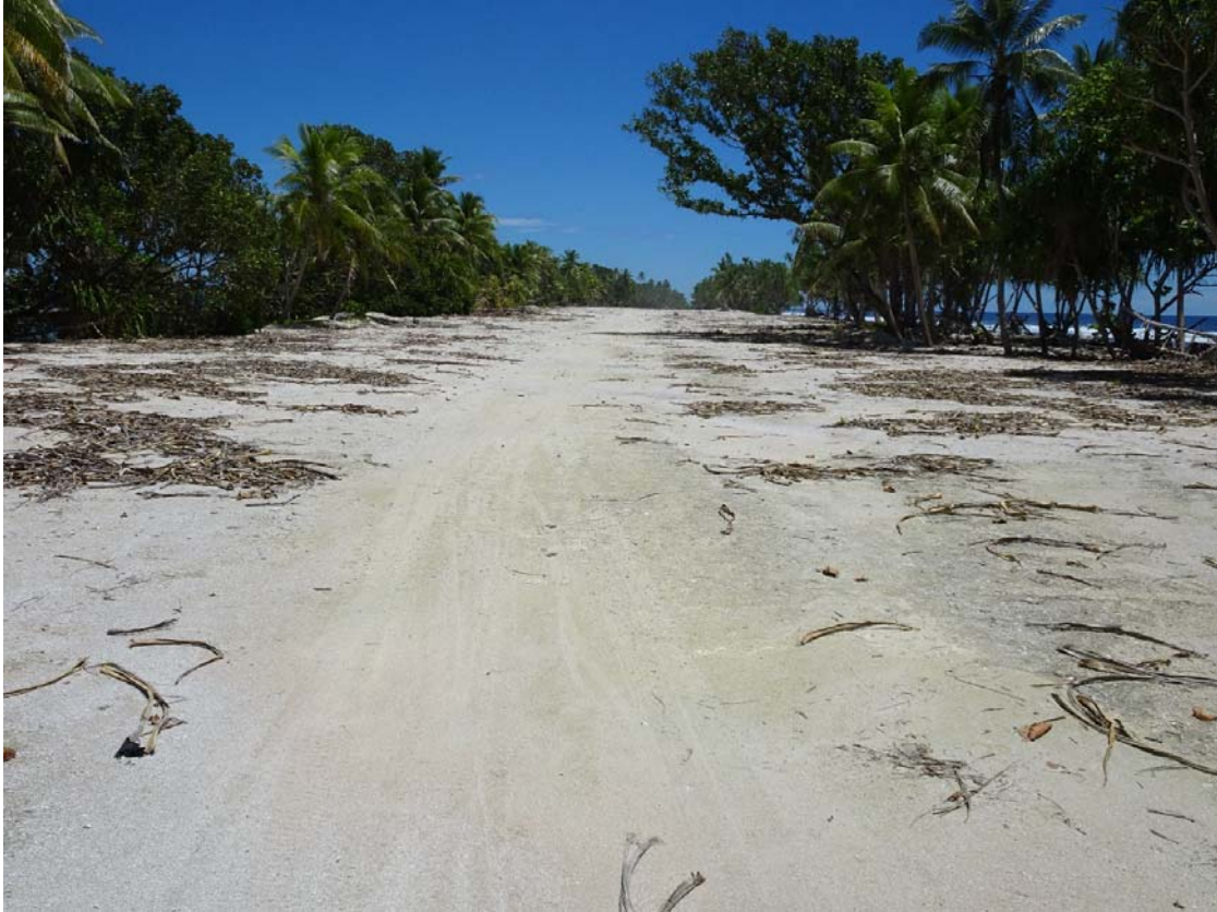
Figure 8. Former borrow pits north of the garbage dump reclaimed in 2015 and infilled with lagoon sediment dredged from Funafuti Lagoon. (Photo: R. Thaman 2016)
