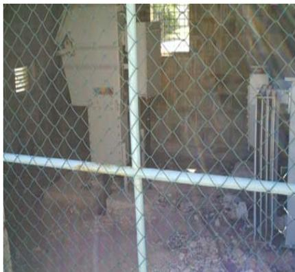
Sub-station #5 at Fisheries, Teone. (No concrete foundation).
