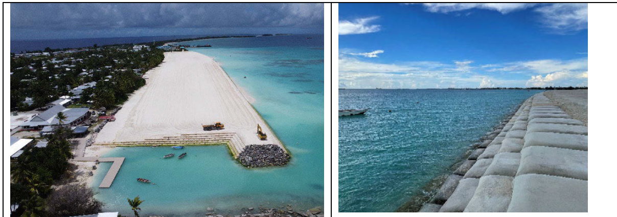
Figure 14-4 Land reclamation undertaken in Tuvalu (source G. Gooley CSIRO). The picture on the left is from TCAP/SPC or GoT.
