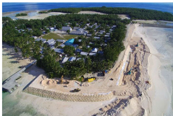
Figure 9-13: Borrow pit filling project at Funafuti (Source: [35])
